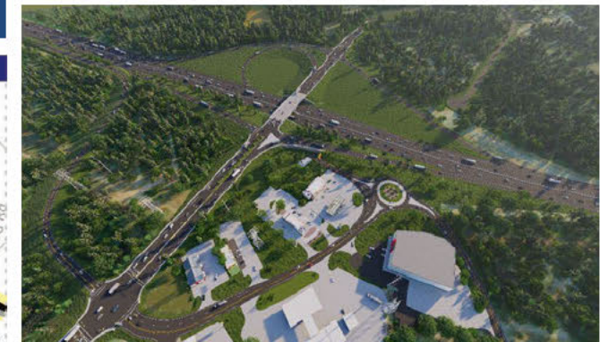
PARCLO at Exit 91 (S-48)
